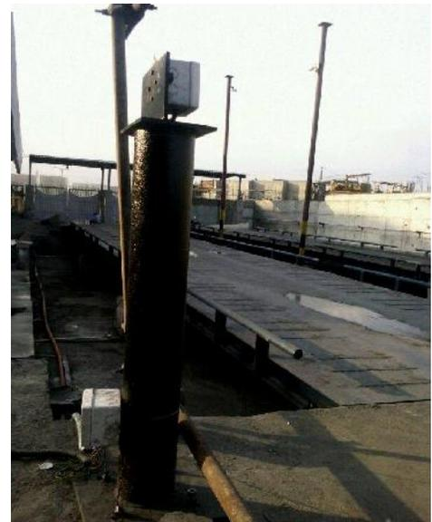
Side View of the RFID Reader installed at entrance of weighbridge
